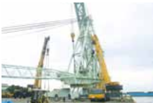
Installation of a crane
