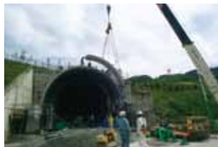
Installation of segment for tunnel
