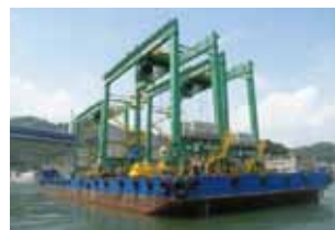
Transportation of structures using barges
