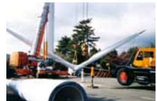
Installation for a wind power station
