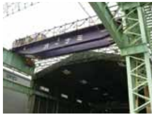
Crane for harbor loading and unloading
